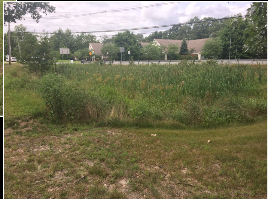
K5 sand lined infiltration basins with volunteer propagules
