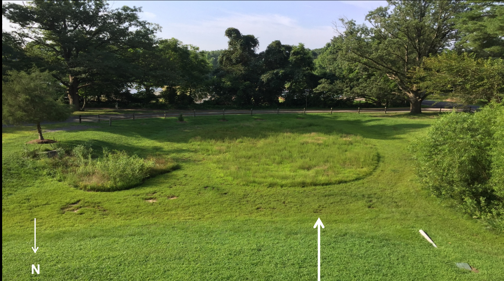
Vegetated Infiltration Basin Pinelands Commission Campus Pemberton Township, NJ
